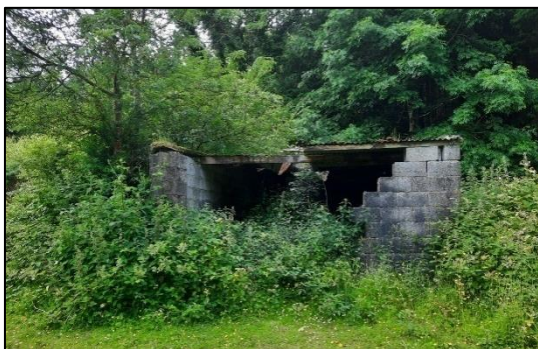
Plate 3-18 Block and Galvanised Sheet Roof Stable Front Exterior
